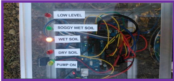
Figure 3.5.2 The soil condition is wet
